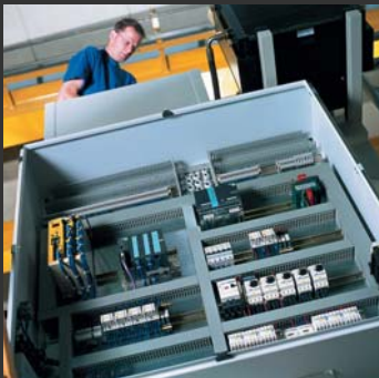
Building the Electrical cabinet
